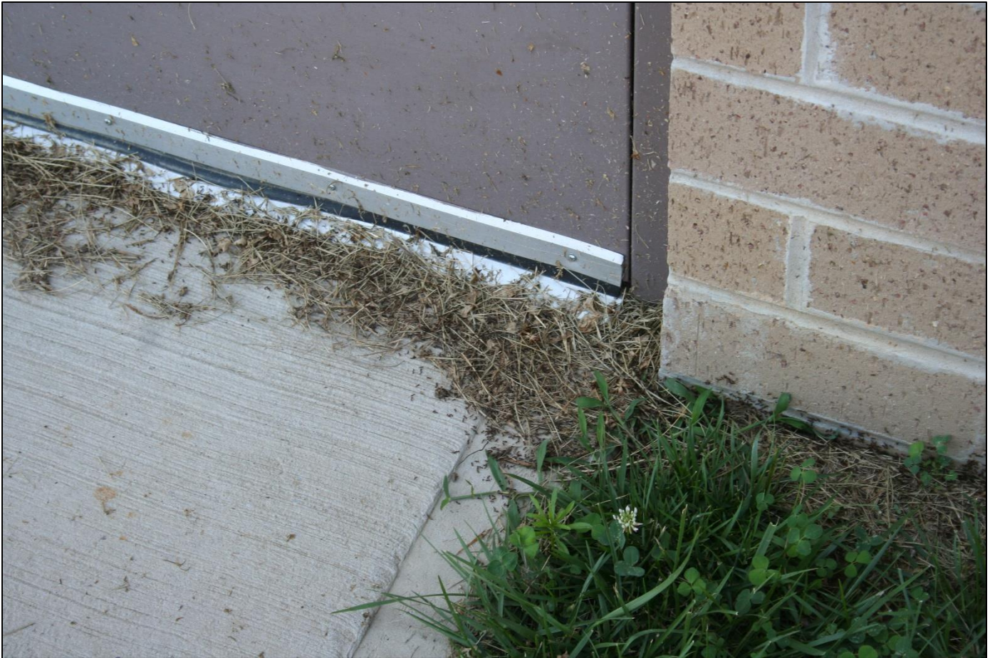
Figure 6. Ants using the foundation base as a guideline can easily follow the edge and enter the structure under the door. Because of their small size, it's difficult to seal ants out of a structure.
