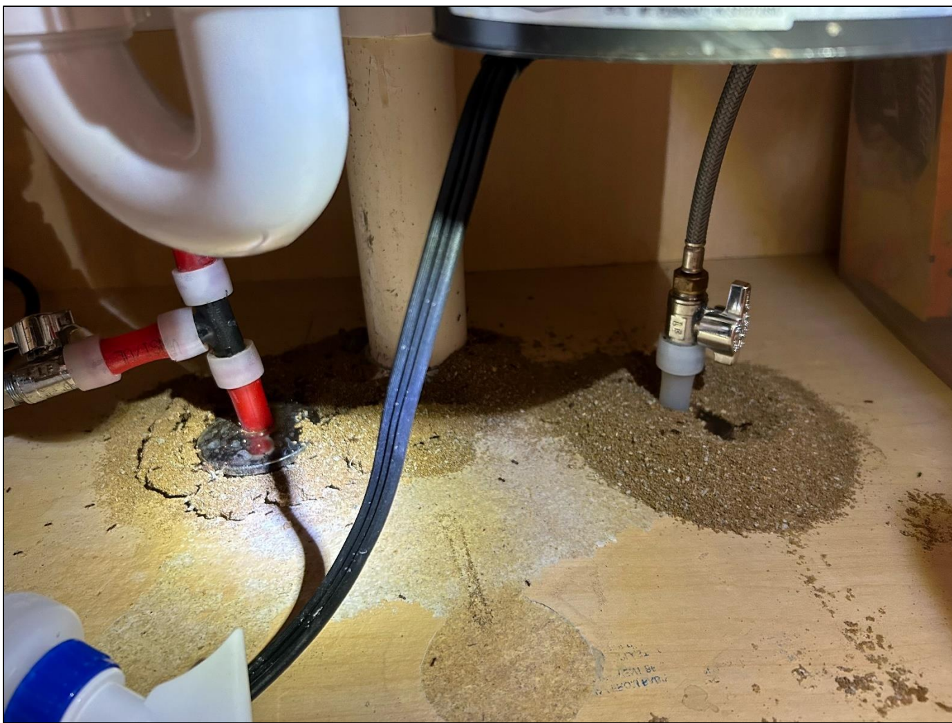
Figure 1. Fire ants have accessed the area under a sink by following the pipe penetration. Note the soil they've brought through the gap. Credit: email submission.
