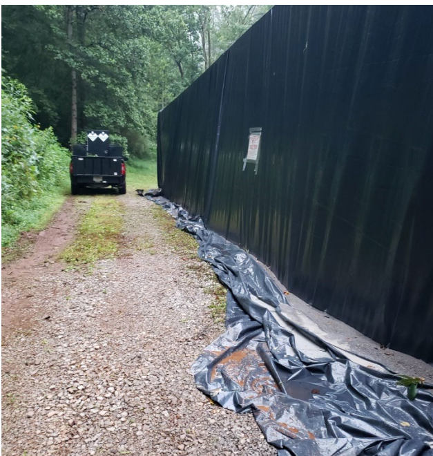
Figure 14. Plastic installed by the family covered the house before fumigation began. Credit: homeowner
