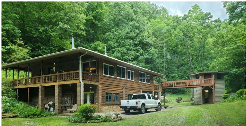
Figure 1. Englewood home with drywood termite infestation on three levels. Credit: John Cook, Massey Services
